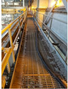
Due to the span of the facility the horizontal overhead crane has to serve the system has been designed allowing for up to 22.5 metres of flexible hose to be attached to any hose connection. Two further vertical pipe extensions have been provided one to each for the air intake filter areas for cleaning purposes.
