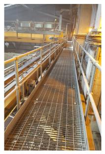
The second application is on the ground floor of the facility beneath the two boilers where there are four platforms, each of these have been provided with a simple pipe work system provided with a vacuum relief valve. At ground level another industrial vacuum cleaning machine has been provided, for this application of one operator using a 51 mm bore flexible hose and tool BVC Centurion Ti80 industrial vacuum cleaning machine powered by a 7.5 kw motor.
